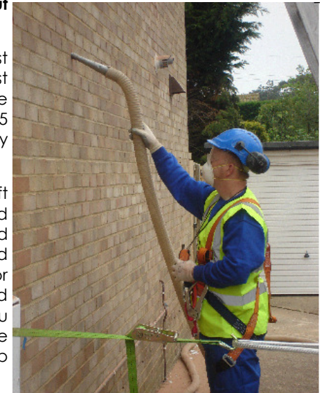
Installing cavity wall insulation
